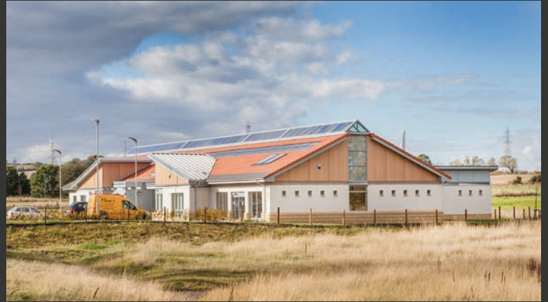
Dual pitched solution with photovoltaic panels, Ormiston, Great Britain
