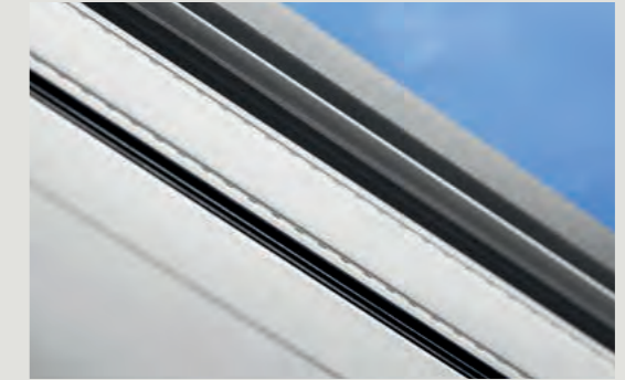
Connection between sash, glazing and outside cladding.
