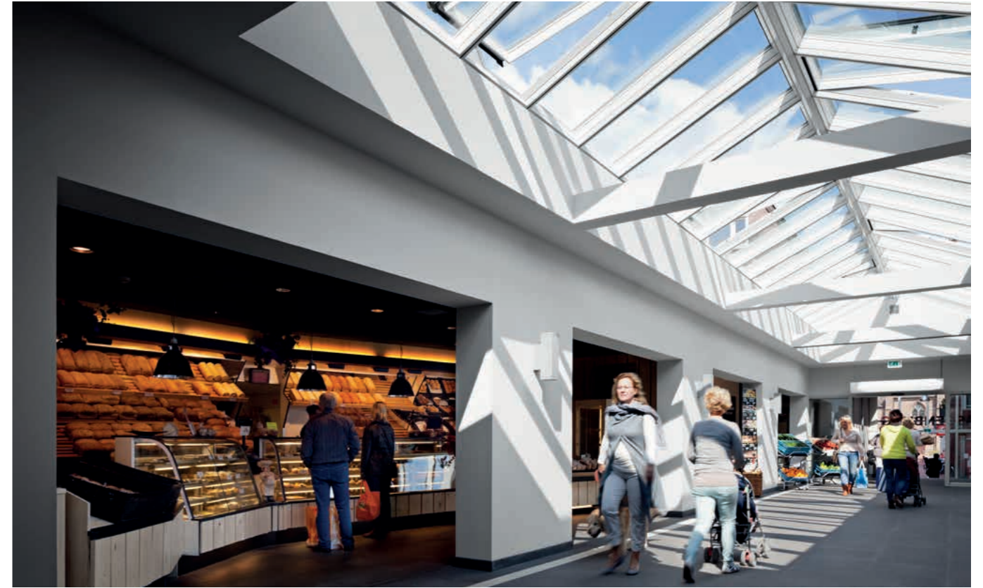
De Assenburg Shopping Mall, Bommel, the Netherlands. 90 modules.
