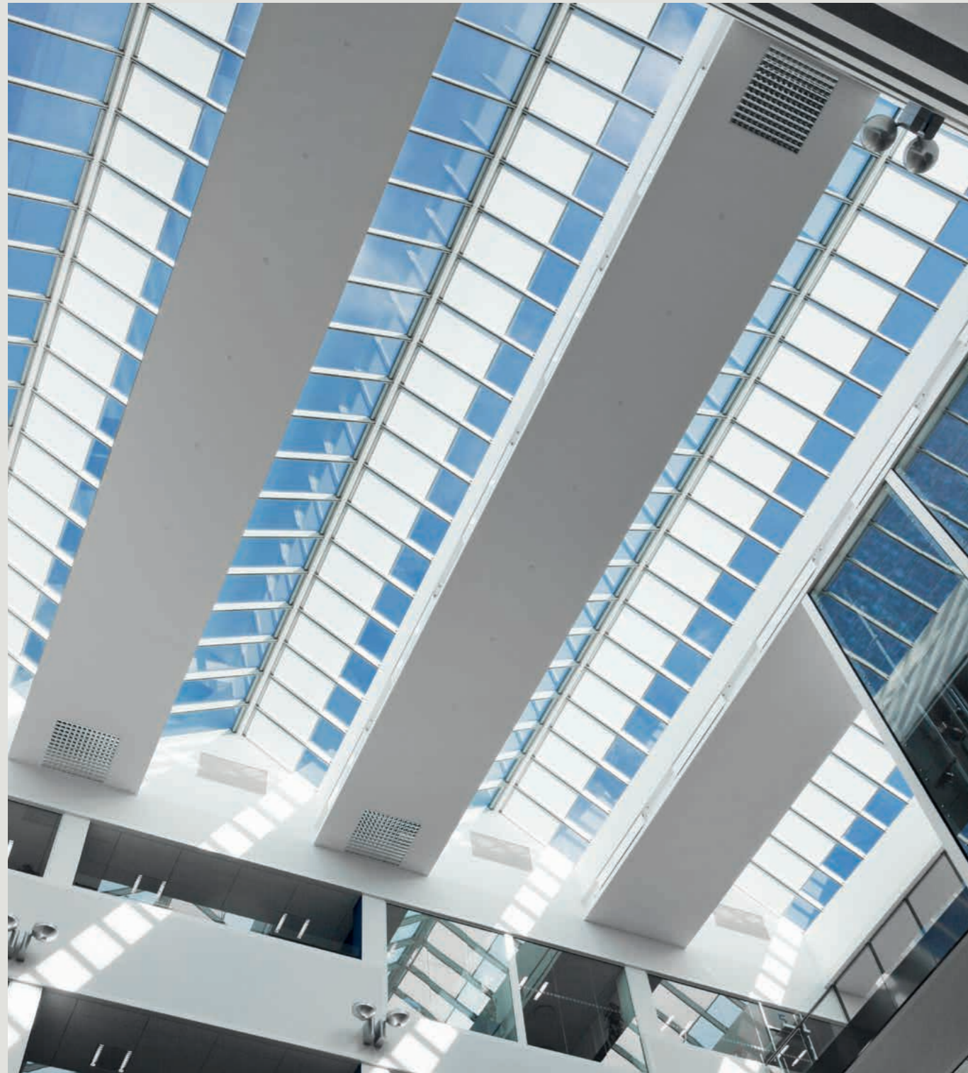
Roller blinds on south facing modules in Siemens Head Office, Ballerup, Denmark
